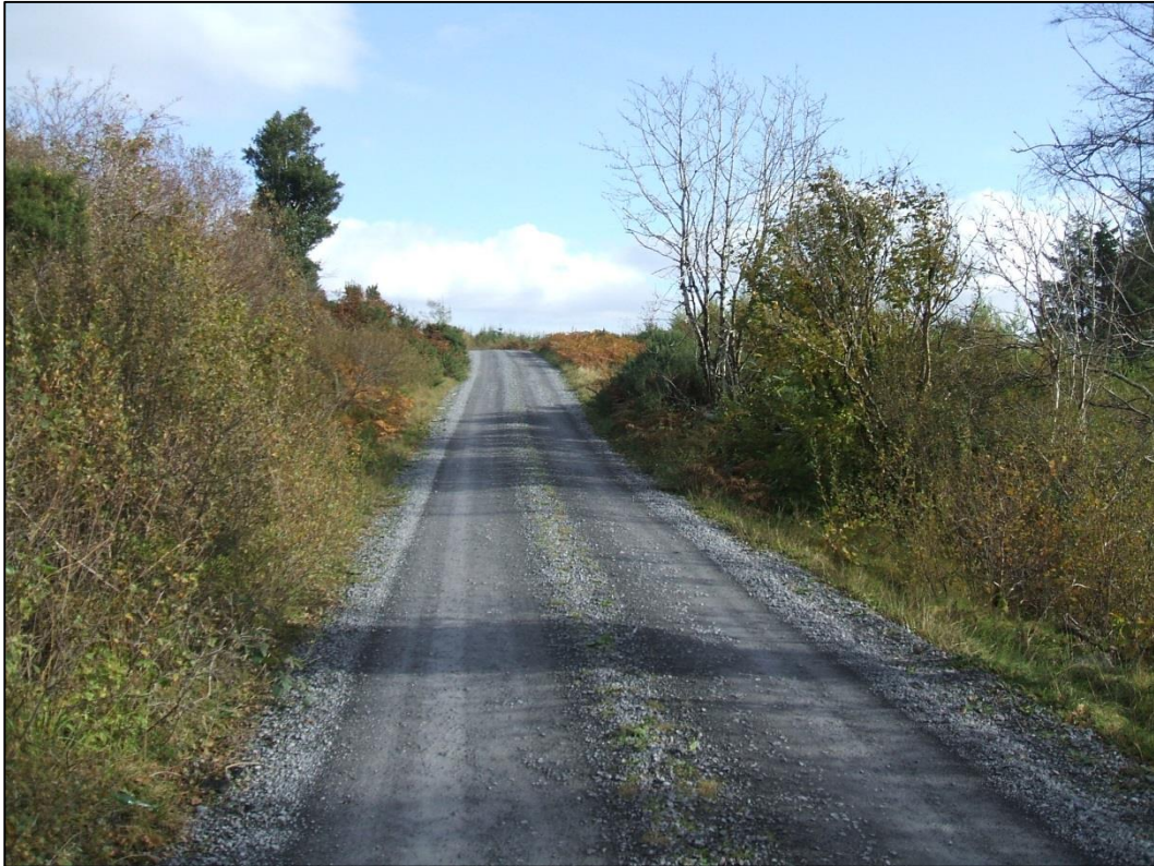
Photo 3 Example of an existing access road on site
