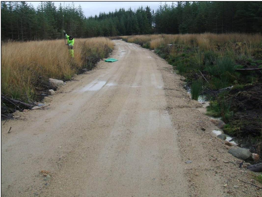
Photo 4 Example of an existing floating access road on site
