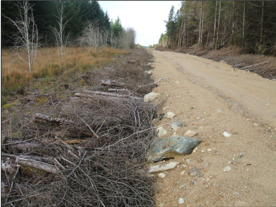
Photo 5 Example of make-up of an existing floating access road on site
